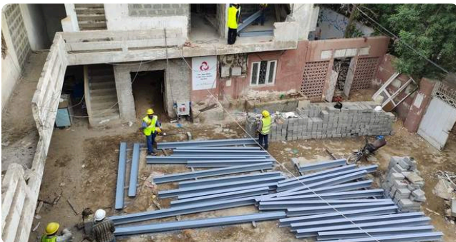
Building strengthening with steel beams
