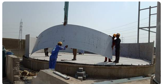
Tank shell plate erection
