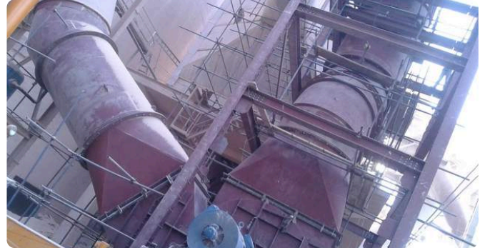
Cyclone and fan installation
