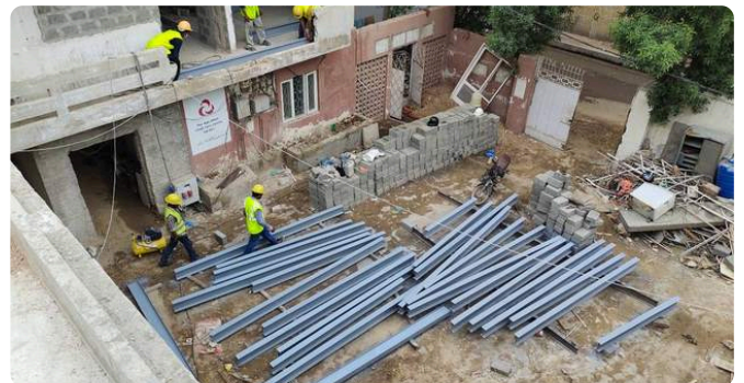
Steel beams placed in existing building
