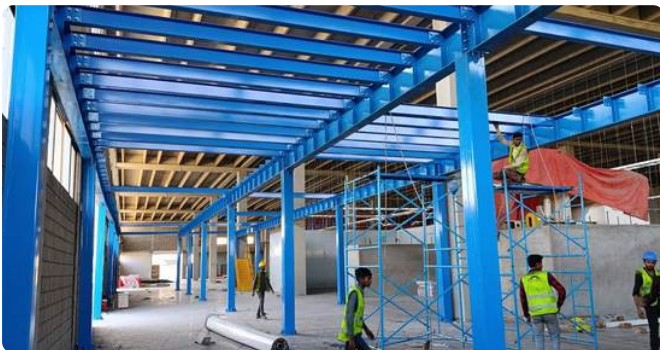
Steel mezzanine structure erection
