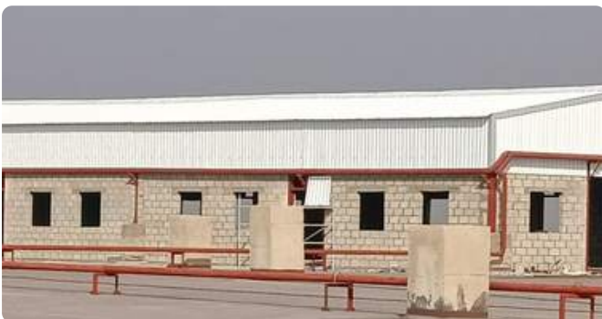
Block-masonry building with steel roof shed
