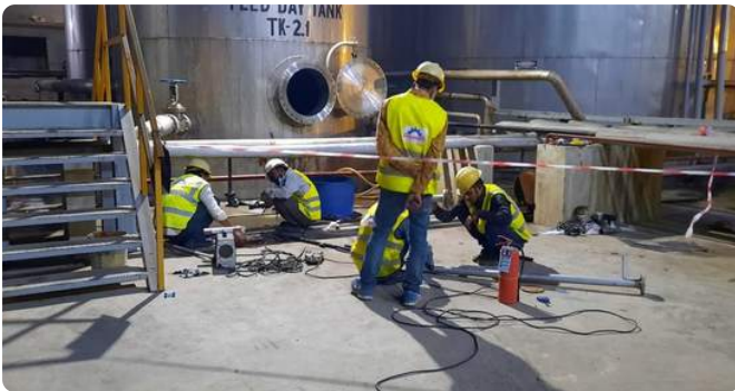
Piping work at Feed Day Tank TK-2.1
