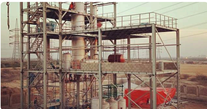
Process plant steel structure
