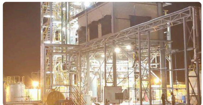
Process plant structure at night
