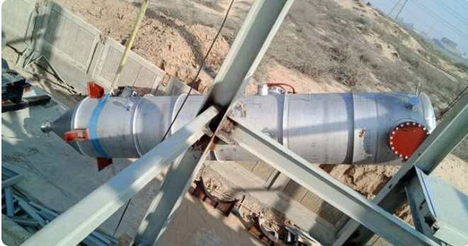
Stainless steel vessel lifted into structure
