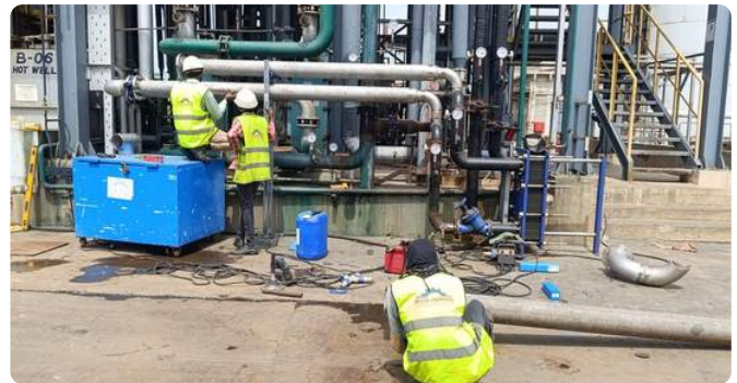
Piping modification at plate heat exchanger
