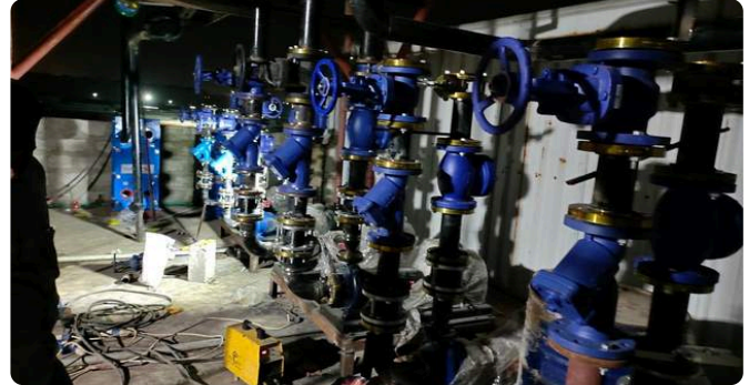
Valve manifold installation
