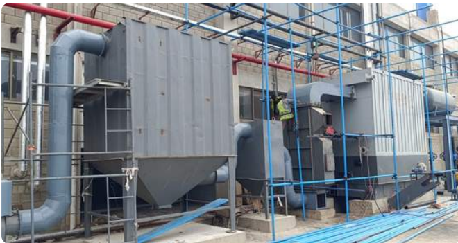
Dust collector and boiler installation
