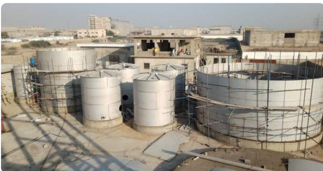
Storage tanks under construction
